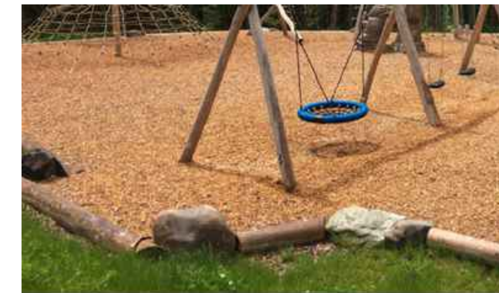
3 TIMBER EDGER WITH NATURAL BOULDER NTS
