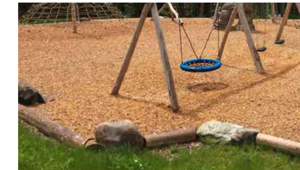
3 TIMBER EDGER WITH NATURAL BOULDER NTS
